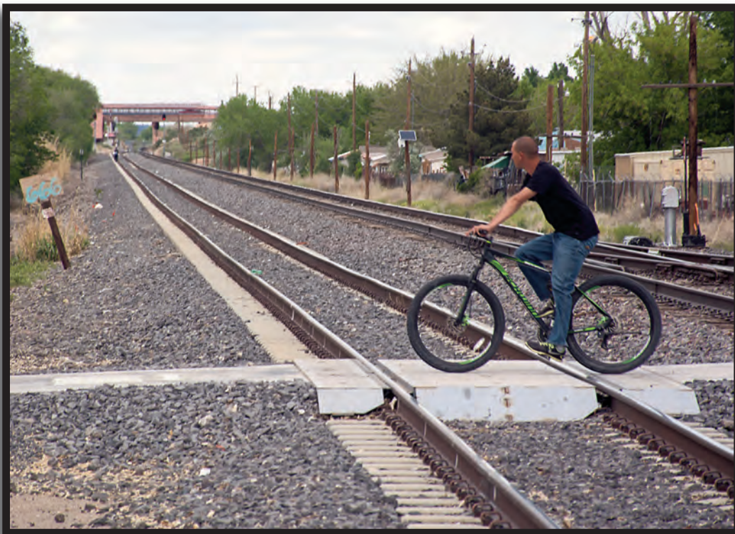
A bicyclist keeps an eye on the rails as he takes advantage of Bernalillo's new pedestrian crossing of the tracks that splits the east part of the town. Flashing lights, bells, and crossing arms that come down protect the crossing when a train approaches.
